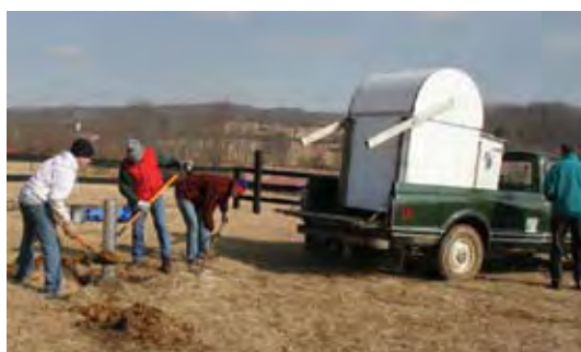
Digging out the pier
