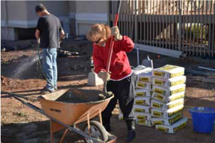
Figure 15: Nancy Mixing Cement for the Pier Base
