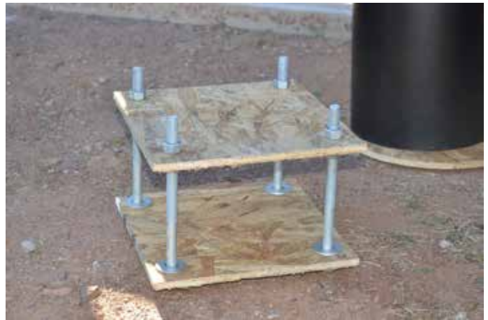
Figure 18: We Built this Jig for the Pier Anchors
