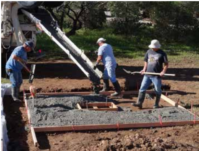
Figure 10: Pouring the Pad
