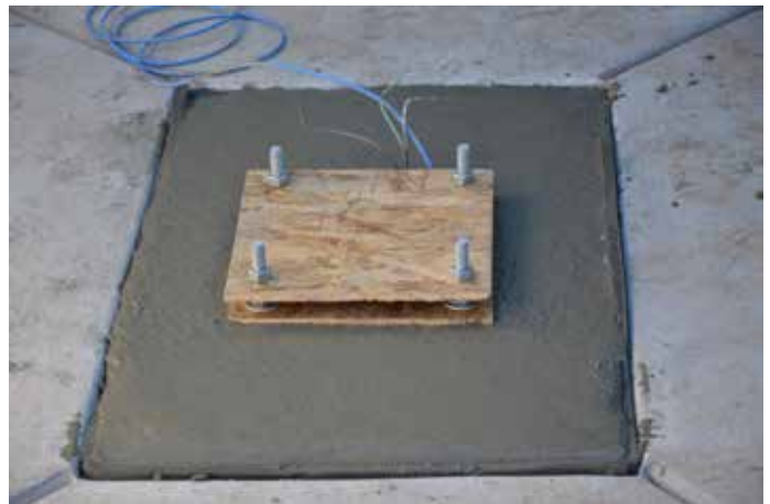
Figure 20: Pier Base Completed on Day One
