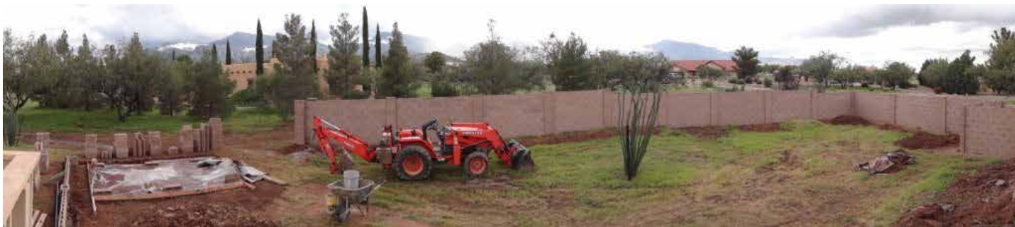
Figure 12: Security Perimeter for the New Area Under Construction
