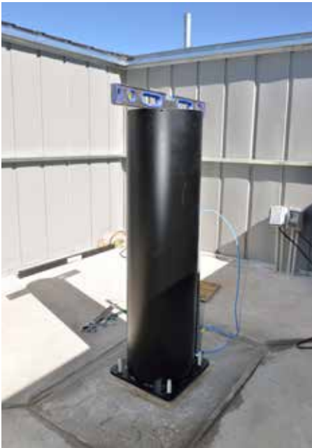
Figure 21: Leveling the Pier with Nuts Above and Below
