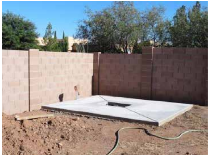
Figure 11: Pad Complete, Ready for the Shed!
