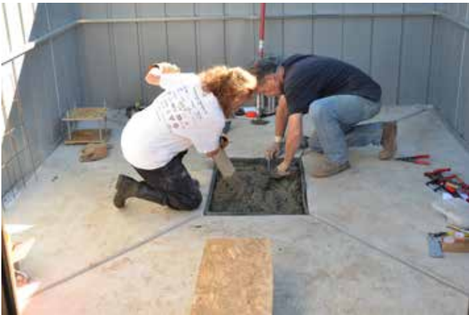
Figure 17: Dave and Nancy Working the Cement
