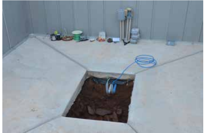
Figure 16: Conduit for Wiring in the Pier Base Hole
