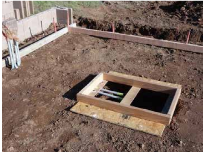
Figure 9: Cutout for the Pier Base. Note the Conduit
