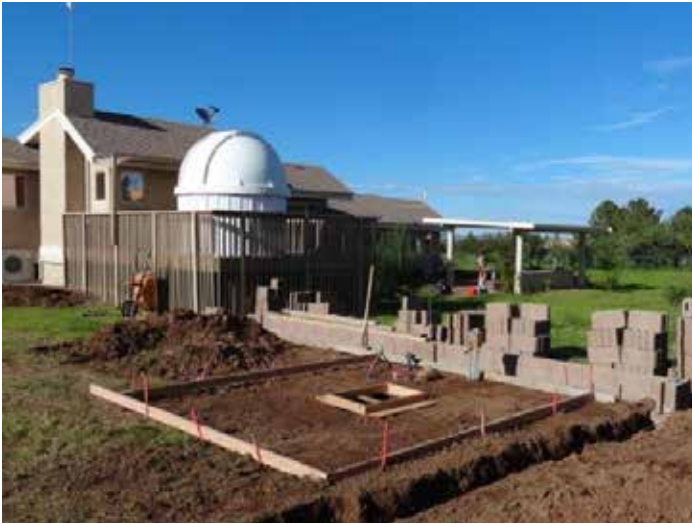
Figure 8: Forms for the Roll-Off Pad
